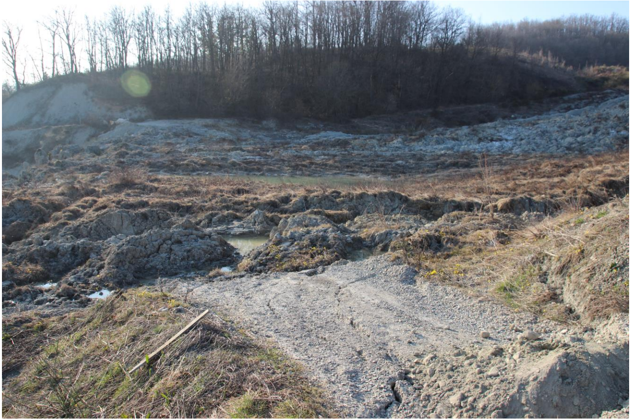
Figure 11. Interruption of the road due to earthflow reactivation.
